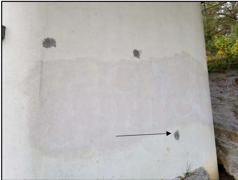
Photograph 10: View of gray cementitious material located at isolated areas on the bents and abutment 2. Bent 1 is pictured in this photo (None Detected).
