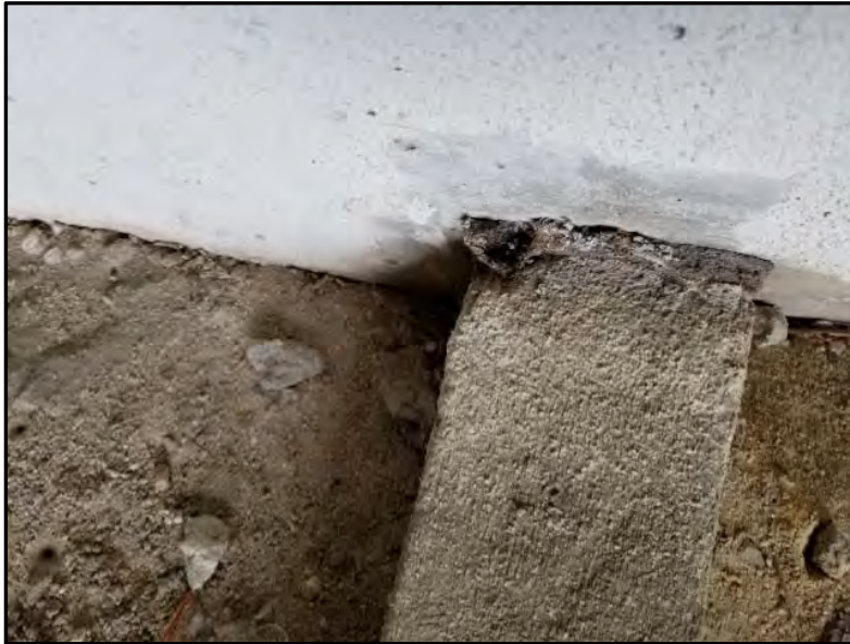
Photograph 11: View of expansion joint sampling point at the interface of the wing wall and the abutment wall (None Detected).
