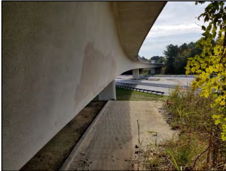
Photograph 1: View of the SC 277 North Bound Bridge over I-77 as seen from the eastern abutment, looking south.
