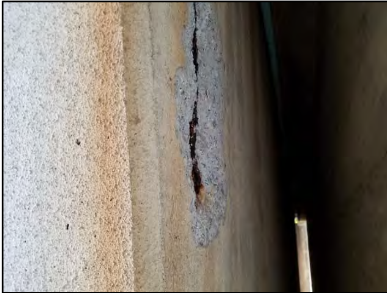
Photograph 9: View of concrete sampling point at the end of the girder adjacent to the abutment wall (None Detected).
