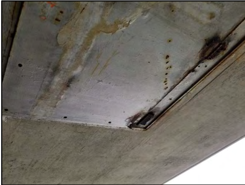
Photograph 17: View of lead based silver paint located on select painted access hatches on the underside of the concrete girder.
