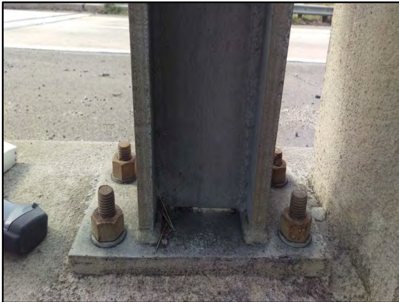
Photograph 16: View of silver painted steel support column located between the bridge girder and the abutment. The silver paint is lead based.
