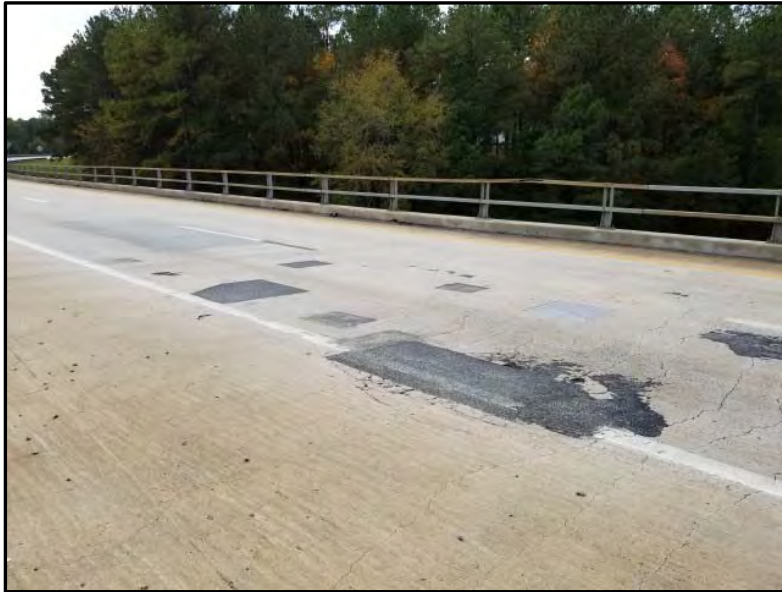
Photograph 13: View of asphalt patching of repaired areas along the bridge deck (None Detected).
