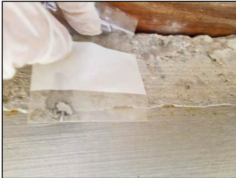
Photograph 8: View of concrete sampling point adjacent to an access hatch on the bottom of the concrete girder (None Detected).
