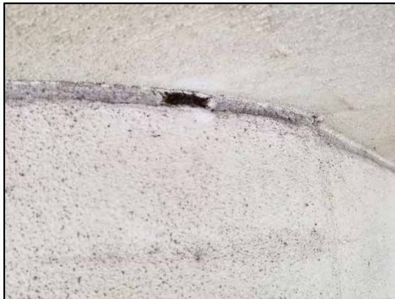
Photograph 6: View of expansion joint sampling point at the top of Bent 3 (None Detected).
