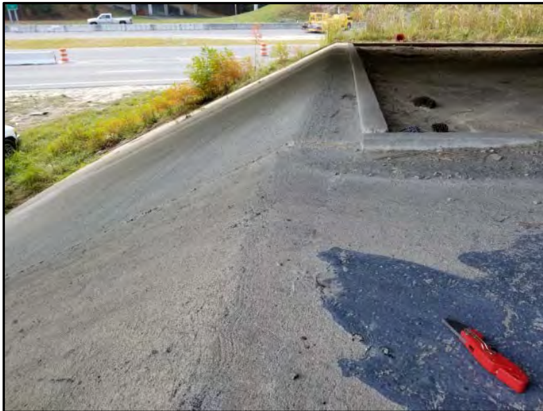
Photograph 12: View of gray mastic sampling point located at the top of the eastern wing wall (None Detected). This material was an isolated spill area at the top of the eastern wing wall.
