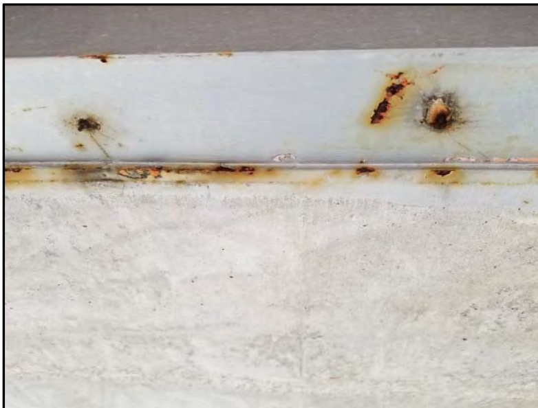
Photograph 18: View of lead based silver paint coated metal access hatch frame located at access hatches on underside of the concrete girder.
