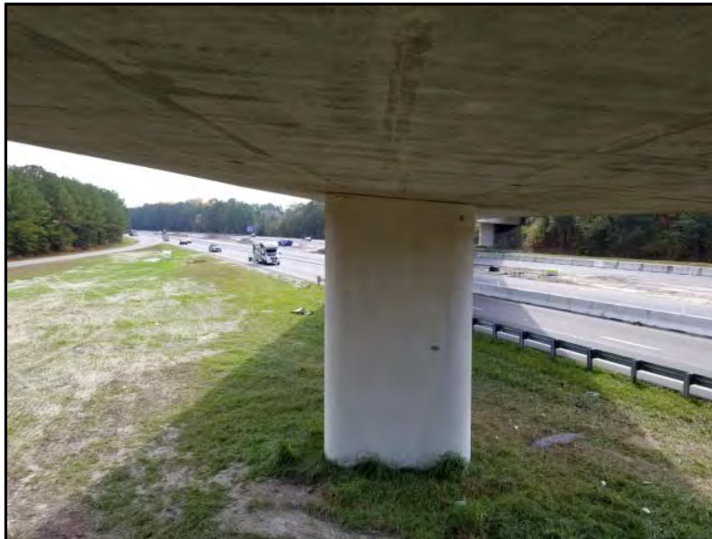
Photograph 2: View of the SC 277 north bound bridge over I-77 as seen from the western abutment, looking northeast.
