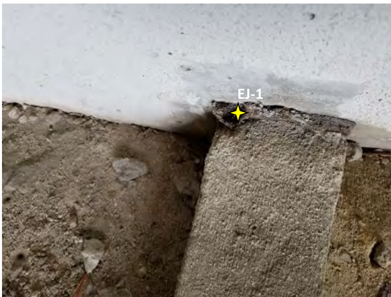
VIEW OF EXPANSION JOINT SAMPLING POINT AT THE INTERFACE OF THE SOUTH ABUTMENT WALL AND WING WALL
