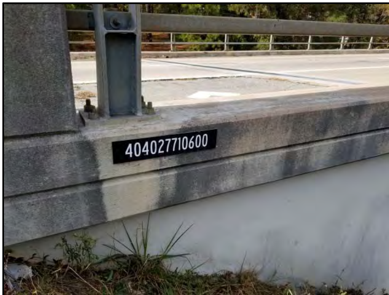
Photograph 4: View of bridge identification number located on the western end of the bridge deck.
