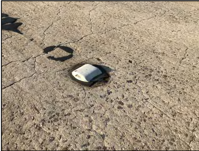
Photograph 15: View of black mastic sampling point associated with reflectors that are located along the center of the concrete bridge roadway (None Detected).
