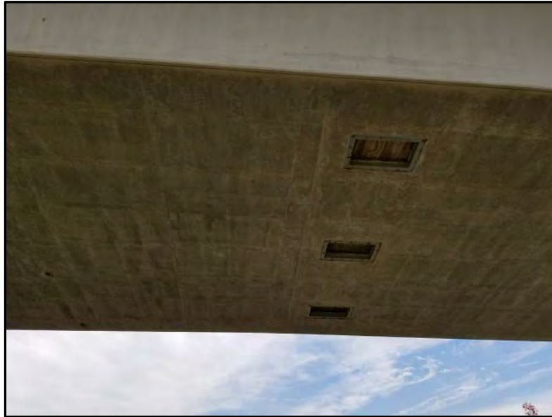
Photograph 7: View of access hatches to the hollow concrete box girder. The silver painted metal access hatch frames and access hatches are coated with Lead Based Paint.
