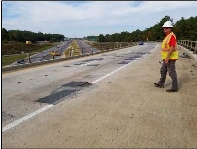
Photograph 3: View of the concrete bridge deck roadway, looking north.
